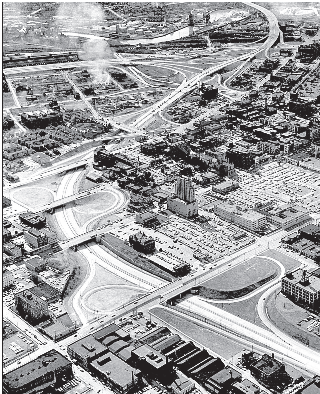
An empty Inner Belt Freeway in 1961, weeks before it opened. The highway would sunder some of Cleveland's oldest neighborhoods, in the name of progress.
