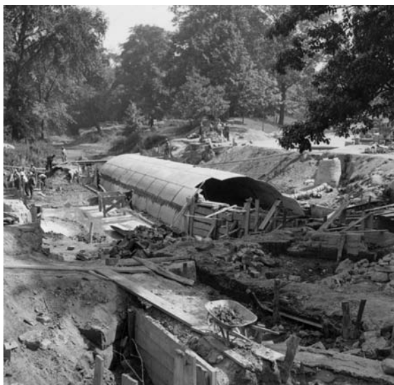
Construction of a Doan Brook tunnel structure, circa 1930.
