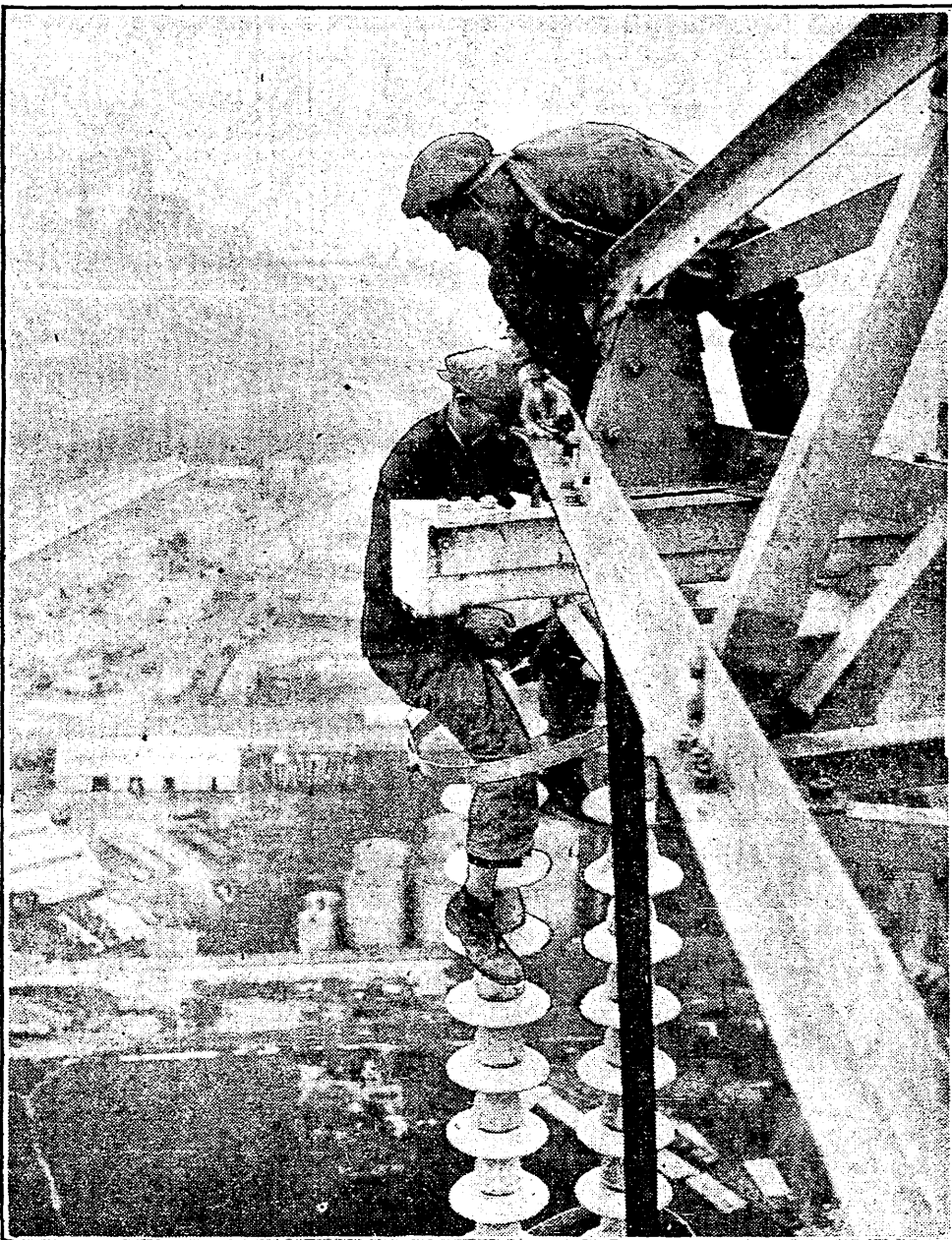
THRILLS IN EARNING A LIVING. These human flies are shown at work on the Thames power transmission tower near London, England. The tower is 487 feet high, the highest in Europe. They are repairing insulator at the top of the tower. (This is the last of the series of pictures which appeared on the Picture Page depicting "Thrills in Earning a Living.")
